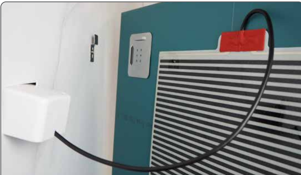
Ensure the demister is wired into a suitable junction box and mount the mirror according to the instructions provided with the mirror.
