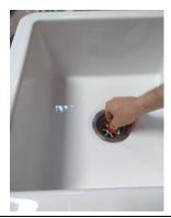
6. Place the sink into the benchtop, wipe away excess silicone, and leave to cure for 24 hours before use
