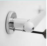
11. Repeat until four screws are securing the wall plate.
