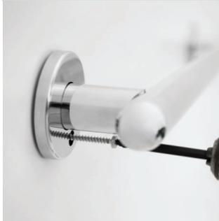
15. Push flange cover over wall plate and insert flange button.
